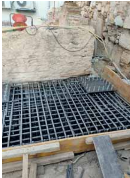
Fig. 15 and Fig. 16: Two views of the completed formwork, after the installation of the metal reinforcement, before being filled with cement. This massive iron and concrete structure is closely surrounded by ancient structures. 2020
