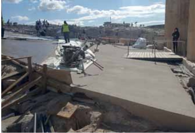
Fig. 3: The area in front of the east front of the Propylaea, in the process of being paved with reinforced concrete, covering over the face of the living rock, October 29, 2020. View from the top of the east front of the Propylaea.
