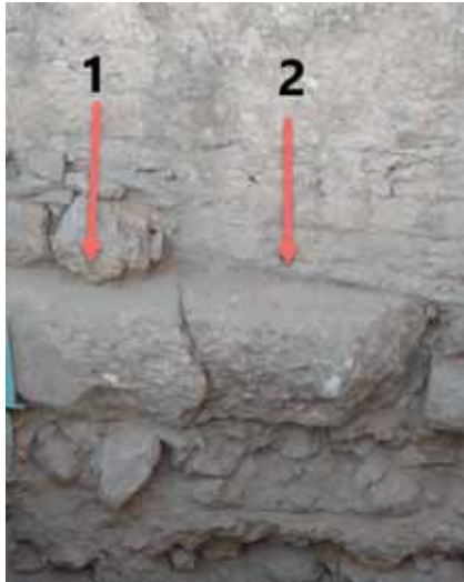
Fig. 12: The red arrows indicate the projecting parts of a poros block, projecting from the wall of a Byzantine cistern, into which parts of the original poros ashlar masonry had been incorporated in a remote past. 2020
