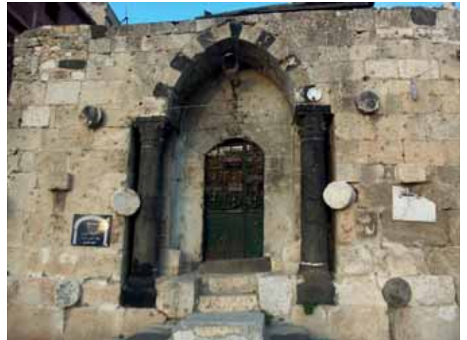
Fig. 7: Al-Qiqan Mosque from the Mamluk era, Stone nails appear in the main façade to support the stone building. Photo: Louay Dakhel, 2018
