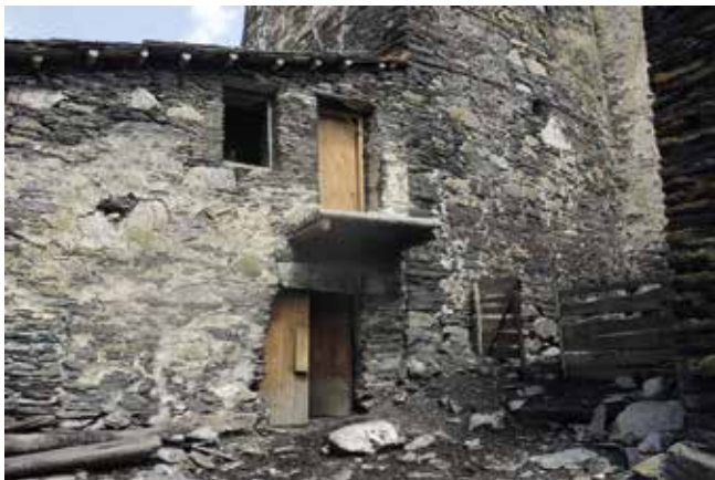
Fig. 8: Poor restoration of Historic building. Use of cement mortar. Chazhashi, 2019.
