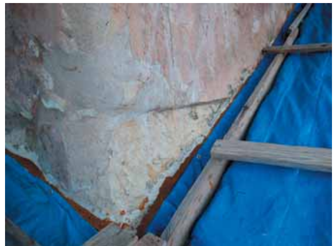
Fig. 5: Open joints between the wall surfaces and the roof construction.
