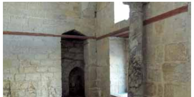
Fig. 8: Citadel Mosque. Horizontal wooden beams appear in its walls to give flexibility to the architectural mass to prevent its collapse due to earthquakes. Photo: Louay Dakhel, 2020
