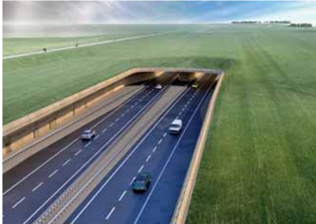
Fig. 3: Image of planned western tunnel entrance. The cutting, through prehistoric cemetery and settlement remains, would be 10–11m deep and 60m wide including its sloped grassed embankments.
