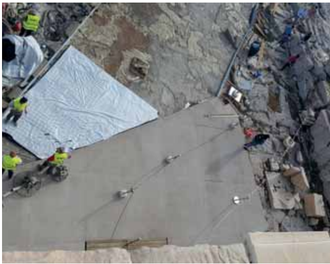
Fig. 3a: The area in front of the east front of the Propylaea, in the process of being paved with reinforced concrete, covering over the face of the living rock, October 29, 2020. View from the northeast corner of the platform. Above left, the west end of the Parthenon.
