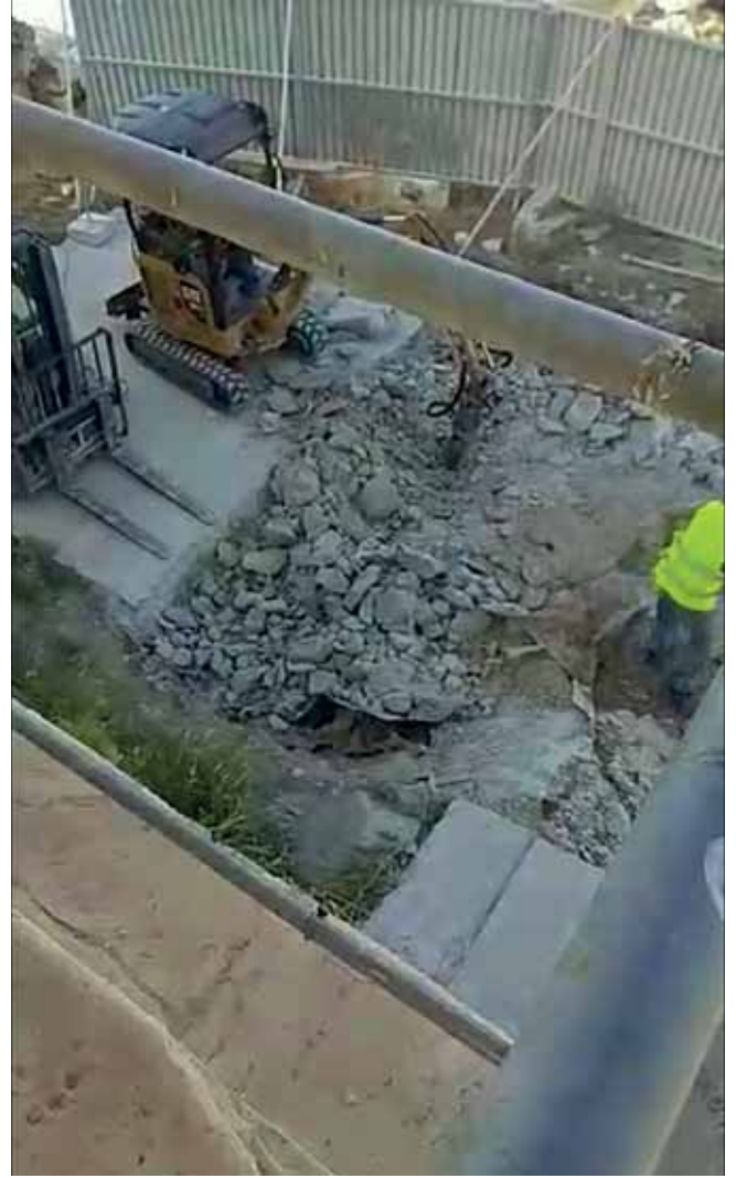
Fig. 4: The area in front of the west front of the Parthenon, view from the west steps of the monument. An impact drill is breaking the massive concrete foundation of the crane that had been erected in this place. Metal panel close the view from the outside.
