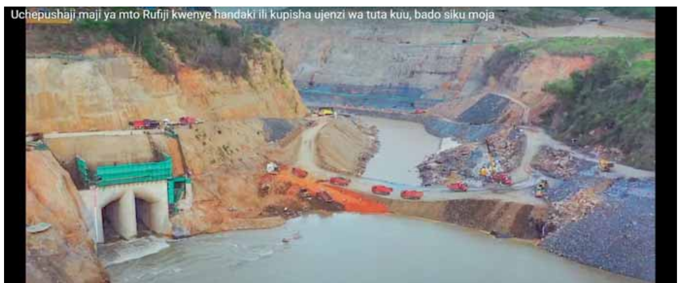
Fig. 1: The Rufiji dam construction site. In the middle, the original river bed, now dammed off, on the left the entrance to the diversion tunnel.
