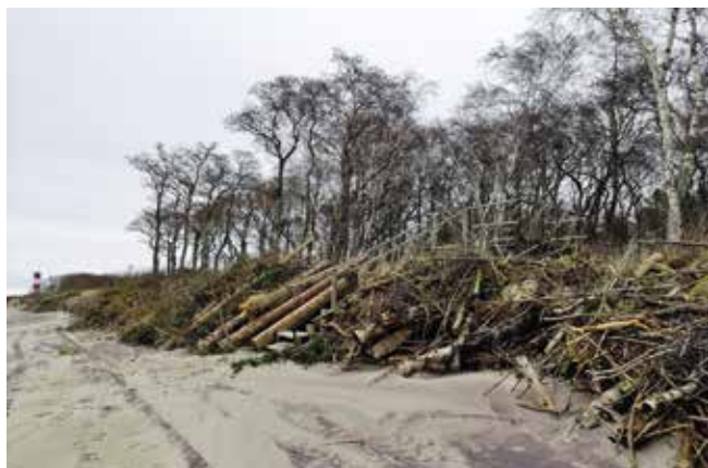
Fig. 5: Repairing the fore-dune with brushwood and poles. Surroundings of the Les-nyoye settlement, 21/02/2019.
